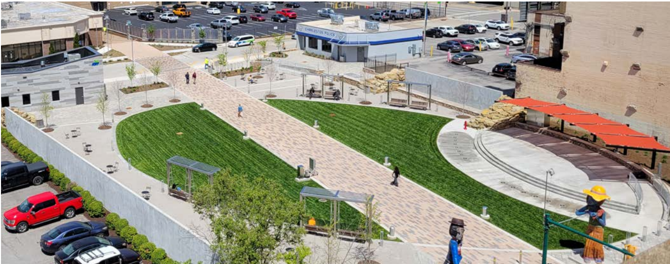
Existing at-grade crosswalk at City Center Station utilizing textured materials, such as pavers, to create a visible and accessible crossing within the transit plaza.
