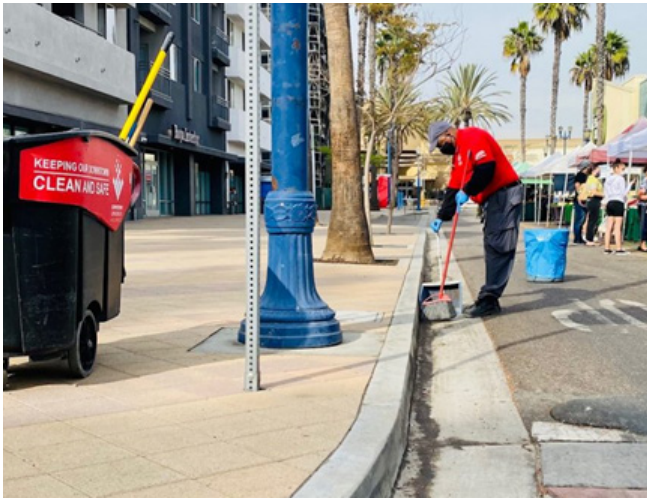
Long Beach Ambassador cleaning the drainage systems.
