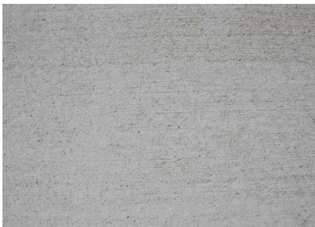
Traditional brushed concrete sidewalks Source: GAI Consultants
