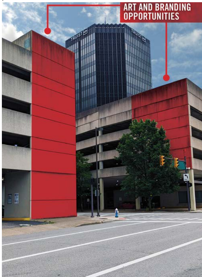
Possible locations for murals on privately owned parking structures.
