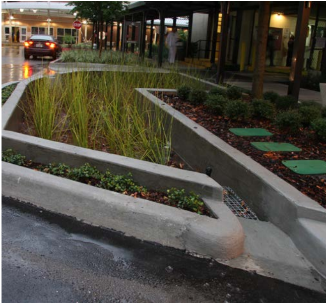
Curb cuts and low vegetation within bump outs for stormwater filtration and clear sight lines.
