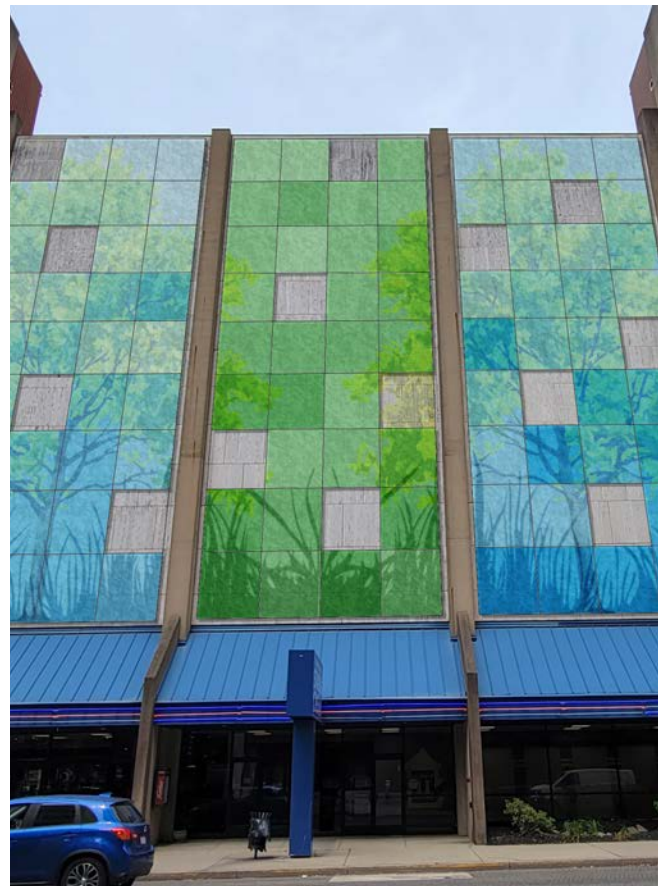
Custom design panels for the movie theater parking garage on Washington Street.
