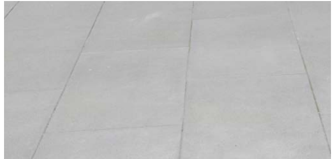
Scoring pattern mimicking the use of pavers in concrete Source: GAI Consultants BRICK PAVERS
