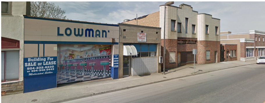
West Washington Street commercial corridor [Source: Google]
