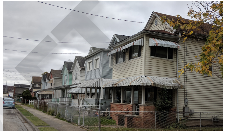
Residential area along 3rd Avenue [Source: GAI, Inc.]
