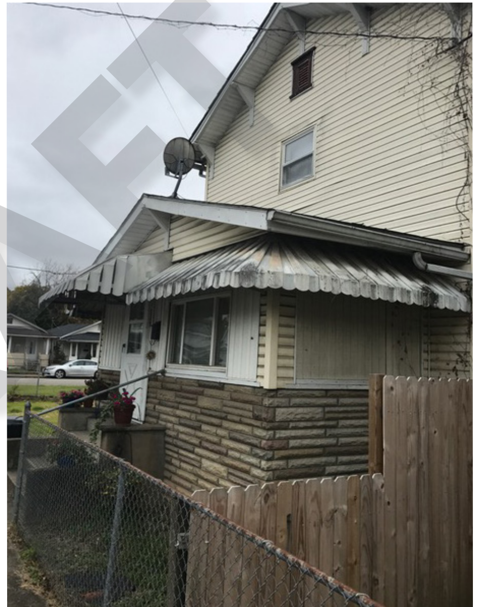
Residential property along Bream Street
