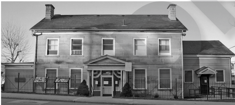
Littlepage mansion [Source: Google]
