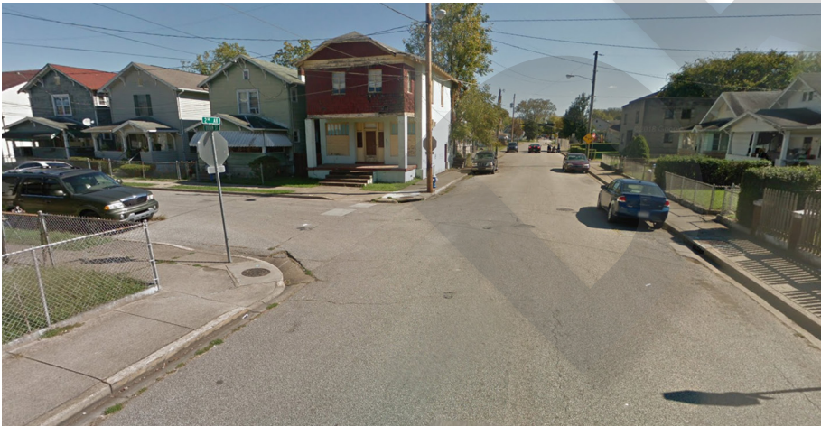
Existing Intersection of Bream Street and 2nd Avenue [Source: Google]
